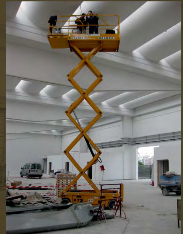
Bari Palese Airport New Civil Protection Headquarter
